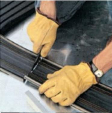
1. Always cut square ends before welding waterstops. Never weld to extruded ends. Use flat work table to create field splices. Work area should be solid and have access to power supply and have jigs and fixtures to aid splicing. Cut ends square, using a razor knife or circular saw equipped with a carbide tipped blade to ensure matching edges.
