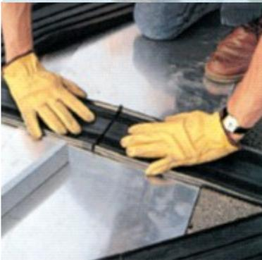
3. Quickly remove **Sireg Welding Blade** and gently press waterstops ends together until they bond (approximately 3 to 5 minutes or cool to touch). Cold water may be sprayed on waterstops to expedite the bond.
