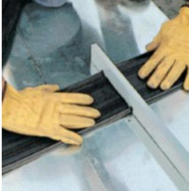
2. Wait that the **Sireg Welding Blade** preheat to the desired temperature ranges. Place the blade between butt ends. Keep waterstops in place until approximately 5mm bead forms on each side of waterstops.
